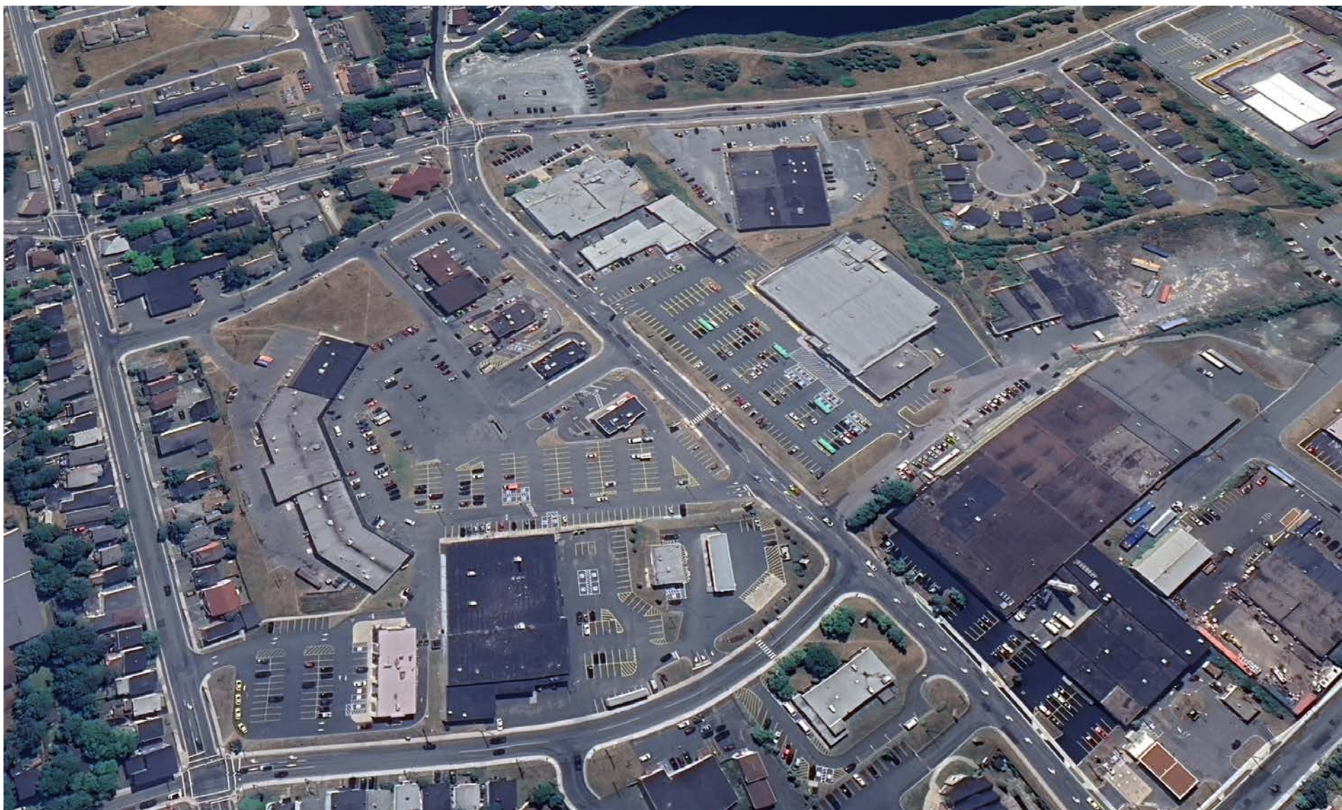
Figure 11. A 2026 aerial view of Ropewalk Lane Mall, showing the existing buildings and parking lots (Google Earth).
